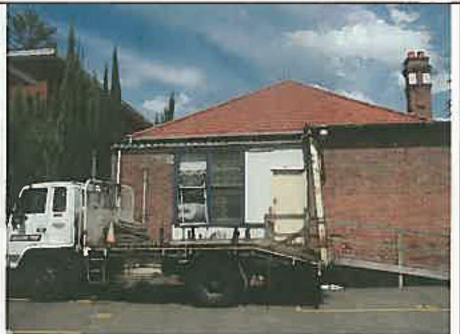
Photo 4, rear of subject building with apartments adjoining
