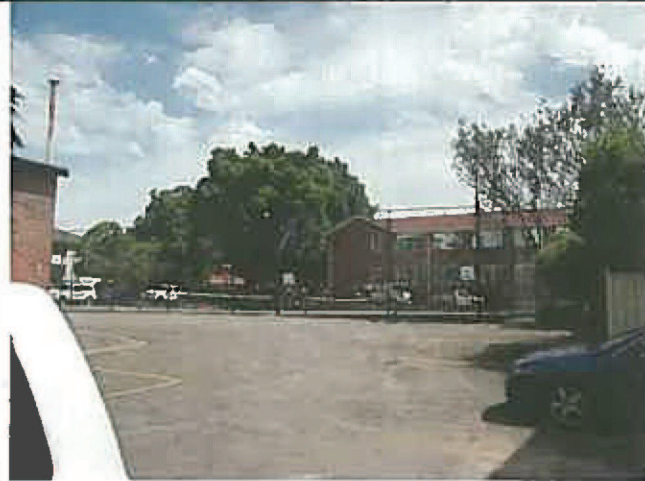
Photo 1, Rear of subject site southwest across tennis courts
