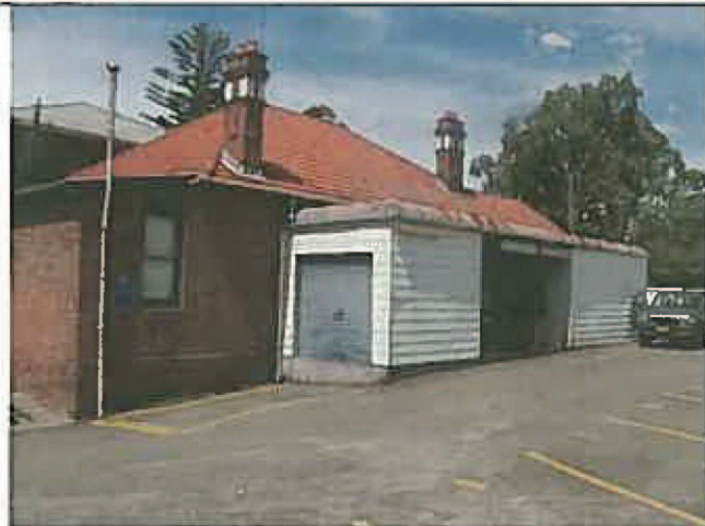
Photo 3, Subject building from tennis court area
