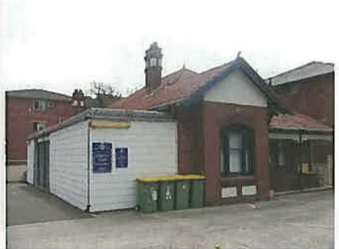
Photo 12, Subject site with surrounding apartments and hard surface.
